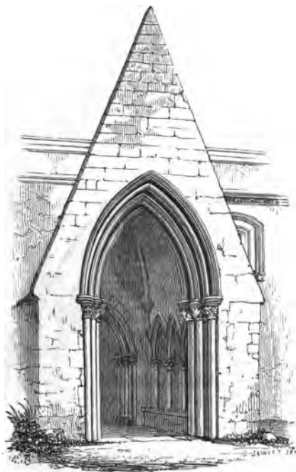
102. Barnack, Northamptonshire, c. 1250.
